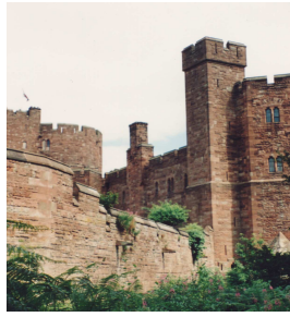
Peckforton Castle and the wall from which I jumped.
